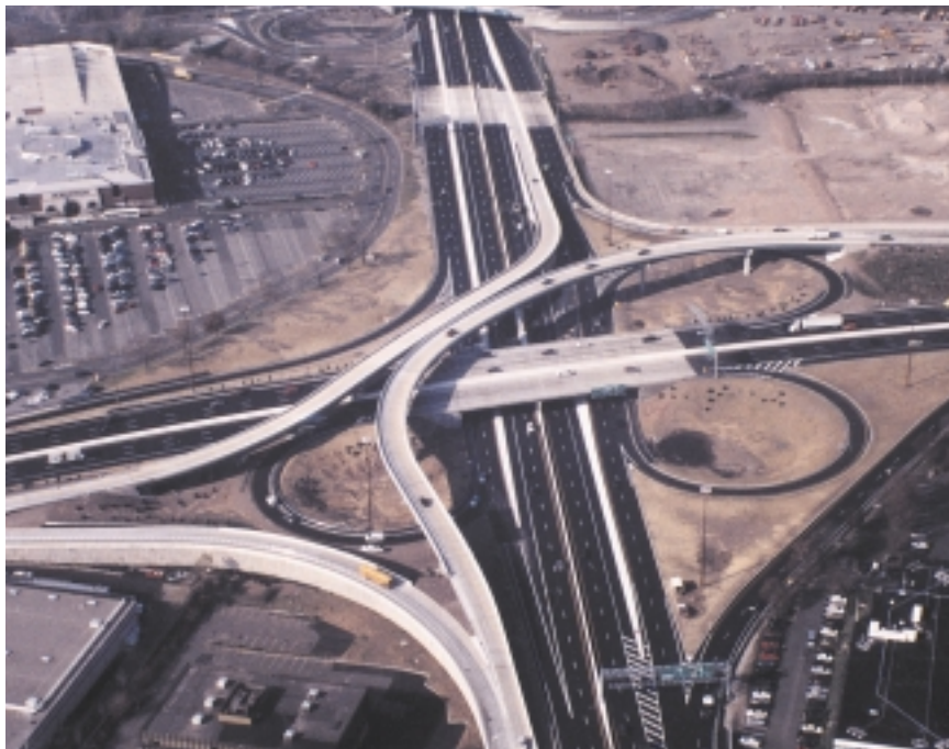
IN CLOVER Route 4 and 17 interchange project set standard for project delivery.
